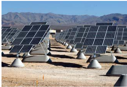
Tracked panels, Nellis Air Force Base, Nevada C.F. ~ 22%
